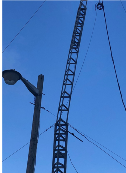
Picture 5: Up-close of Bent Tower
