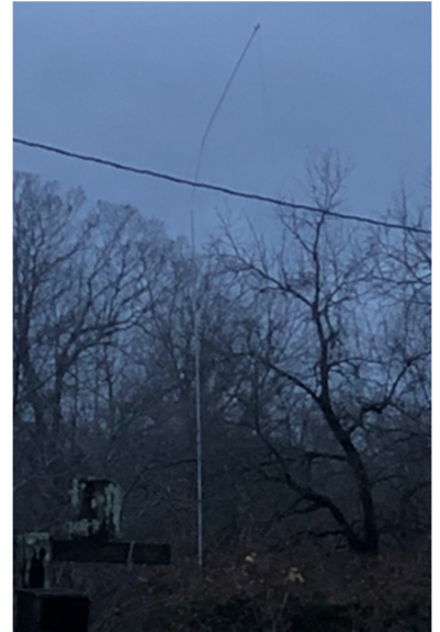
Picture 6: Bent 160m Vertical Antenna
